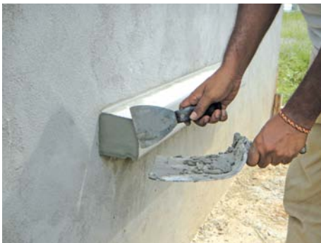
g) Cover both 2 ends of foamcrete cornice with foamcrete cement.
