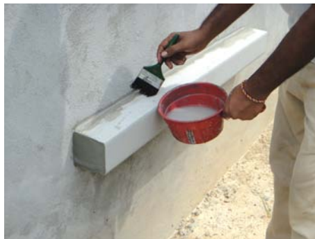
h) Trim foamcrete cornice surface with brush and water.
