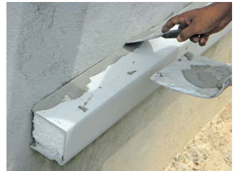
f) Infill foamcrete cement in between gap of foamcrete cornice & wall.
