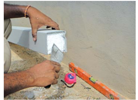
c) Remove polystyrene foam of 2 ends with scraper.
