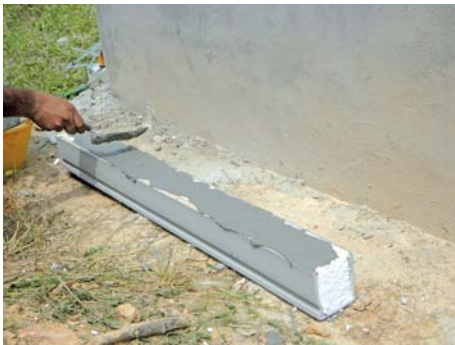
d) Apply foamcrete cement to polystyrene foam surface.
