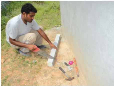
a) Cut foamcrete cornice to required length by using saw.
