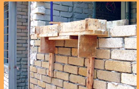
Conventional method (above) of making window sill is labour intensive & time consuming.
